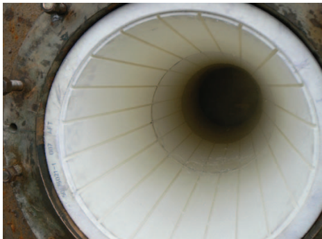
Full form SXL bearing installed in stern tube.
